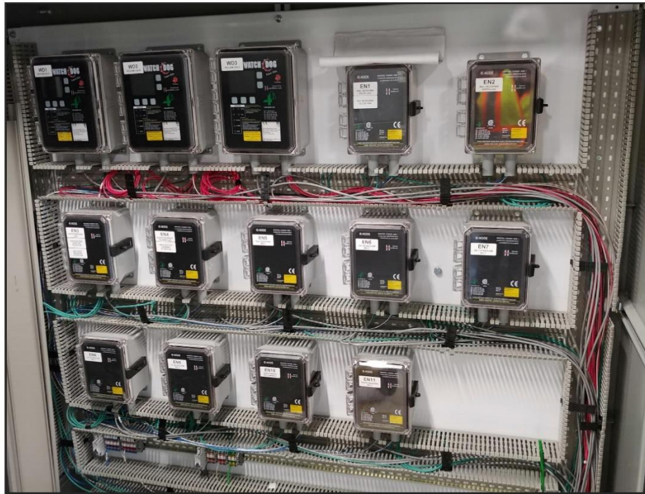
Figure 35: Combination standalone controllers and Industrial Ethernet nodes. (Photo courtesy of 4B Components, Ltd.)
